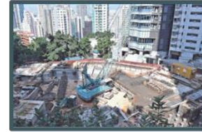
• 8 Castle Road, Mid-Levels (4A-4P Seymour Road)
