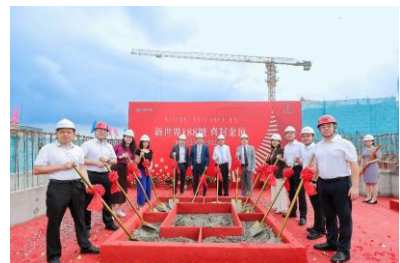
Construction of New World 188 is progressing steadily, with the topping-out of its first-phase residential component, WELL SPRING, marking a new development milestone.
