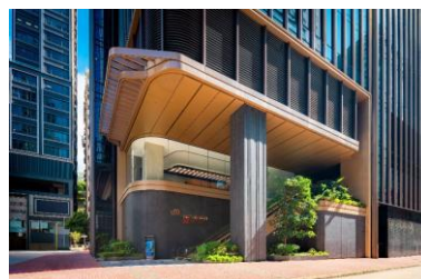
83 Wing Hong Street, the Group's Grade-A office project in Kowloon West, sold over 75 units, representing nearly 80% of the units launched, with an average transaction price of approximately HK$7,500 per square foot.
