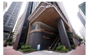
83 Wing Hong Street, a Grade-A office building in Kowloon West, recorded 10 transactions in recent months, exceeding HK$100 million in contracted sales.
